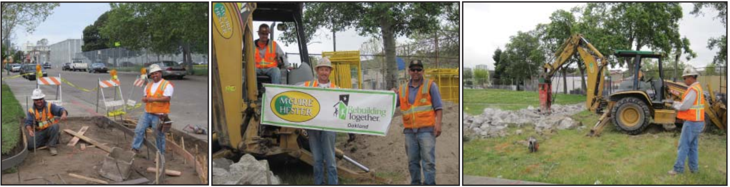
Crew (left to right) Ramon Figueroa, Victoriano Martinez, Jorge Gomez, Dave Burgeno and Milton Vasquez prepare site for the installation of playground equipment
