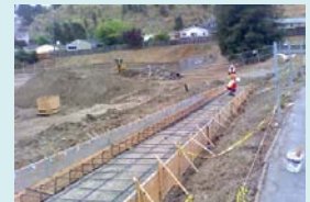
above: 2991 crew laying forms for a concrete walkway and dugout
